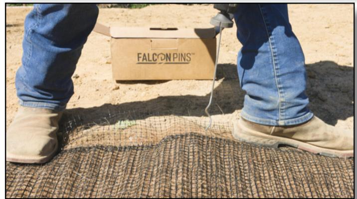
*VMax turf reinforcement mat being installed on a channel application (top right), twistex pins installed with TRMs can have increased system performance and pullout resistance (middle right), twist pins are available in 8" and 12" lengths and two coil configurations designed for hard or soft soil types (lower right).*
