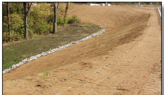
Biodegradable ECBs offer an environmentally-friendly alternative to traditional photodegradable ECBs in high-risk areas.
